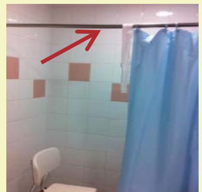
Metal rods that patients used for hanging in toilets
