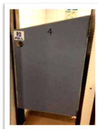
Enhanced toilet cubicle door with anti-ligature design
