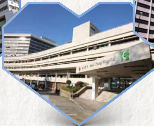
Kwai Chung Hospital
