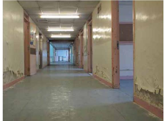
▲ Deteriorated finishing at ward corridor
